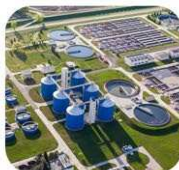
WATER AND WASTE WATER TREATMENT PLANT
